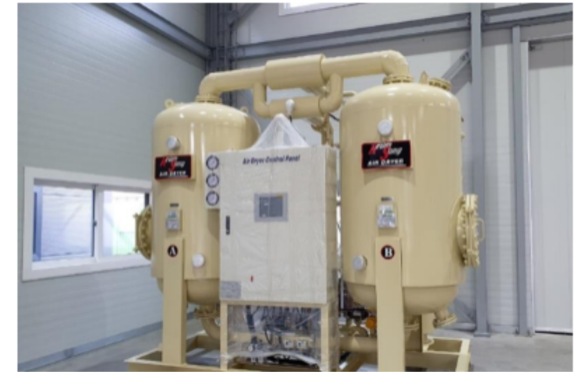
N2 GENERATOR SYSTEM
