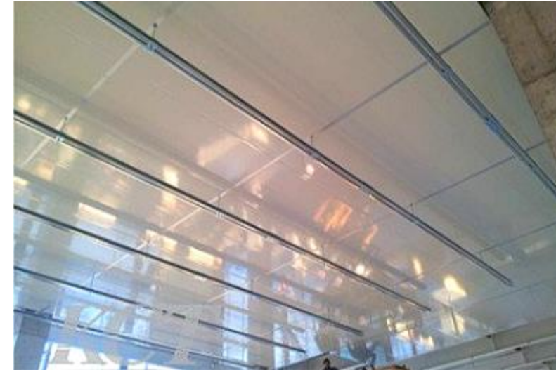
Main & sub C-beam installation
