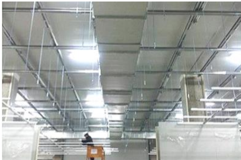
Air conditioning ducts, secondary electrical installation
