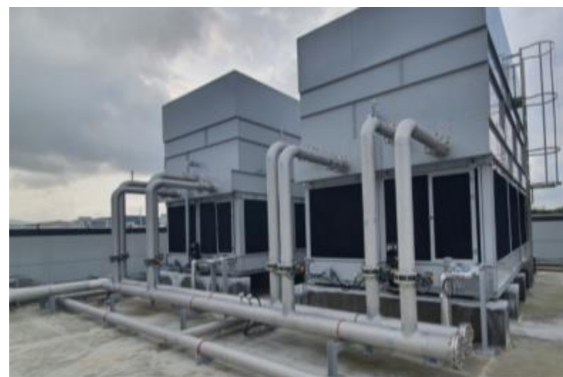
Installation of closed cooling tower
