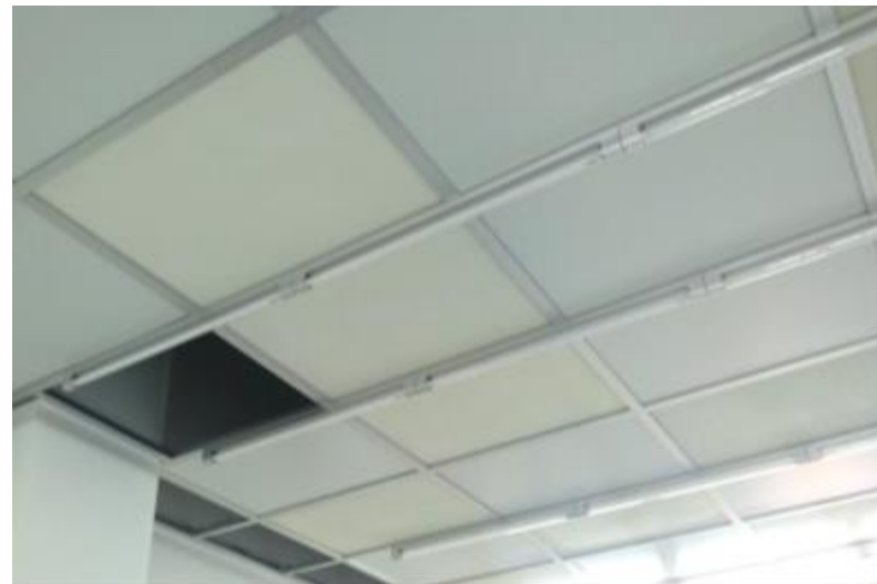
Installation of FFU & TD etc.
