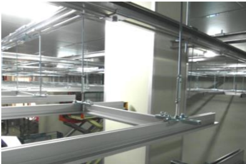
AL mold bar installation
