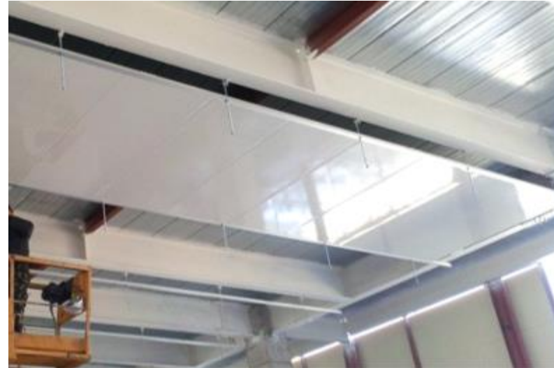
Air conditioning ducts, secondary electrical installation
