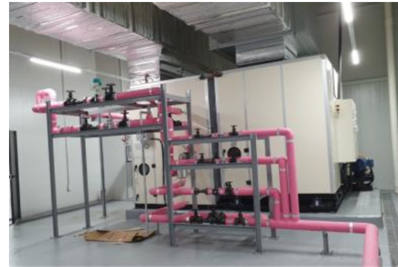
Air conditioner and piping installation
