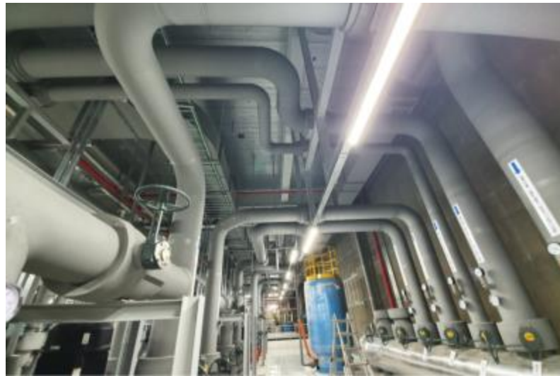
Compressed air piping construction
