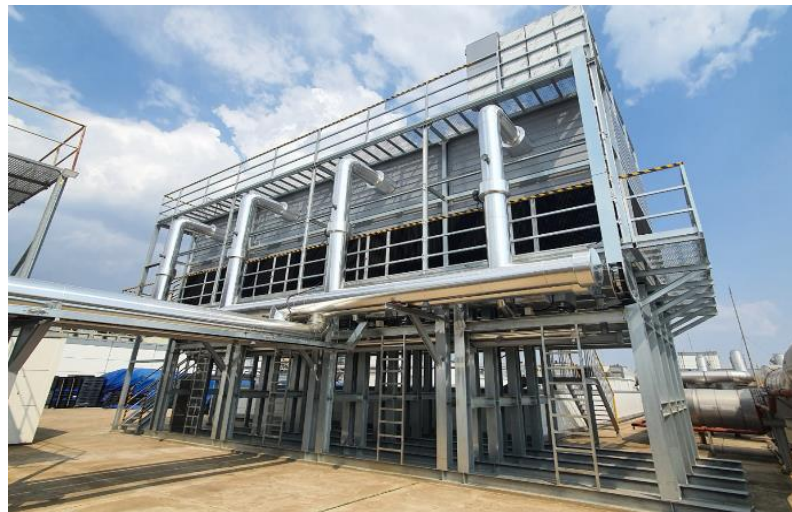
Cooling tower piping construction
