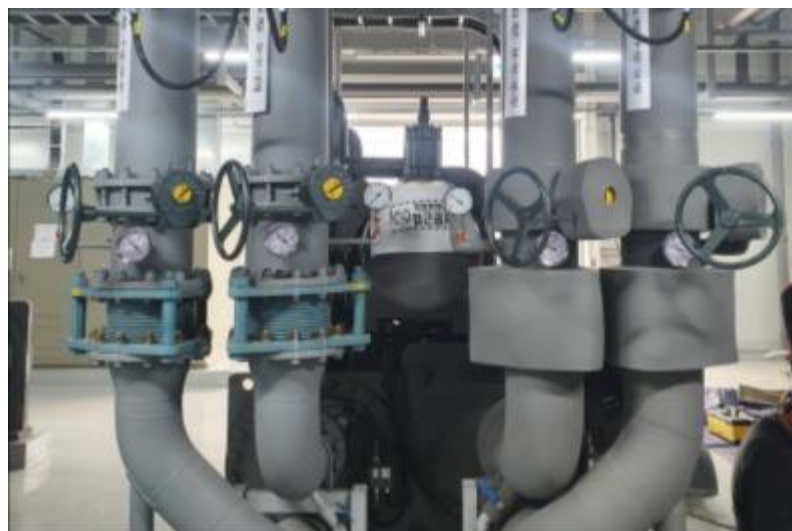
Screw chiller system installation
