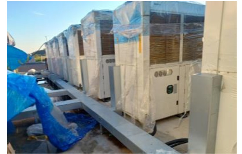
Installation of outdoor unit for air conditioner
